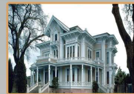
Standalone Access Control: House
